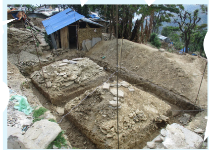
Trench level for foundation ready
