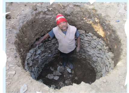
Septic tank construction for toilet
