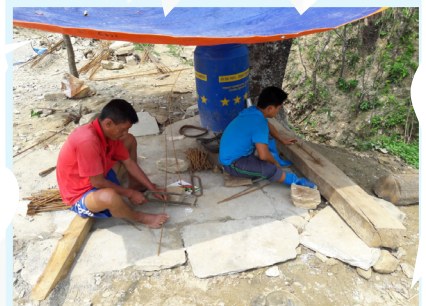
Bending reinforcement for beam
