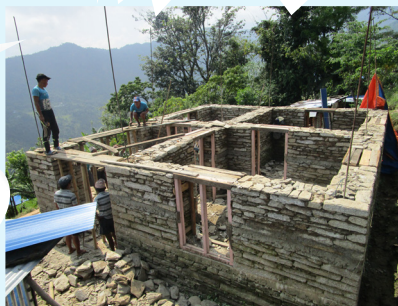
Beam level house construction
