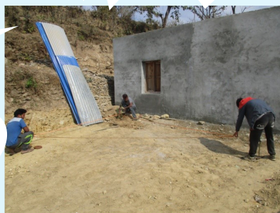
Layout for house construction
